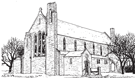
St. Matthew's Anglican Church, 2165 Winnipeg Street
