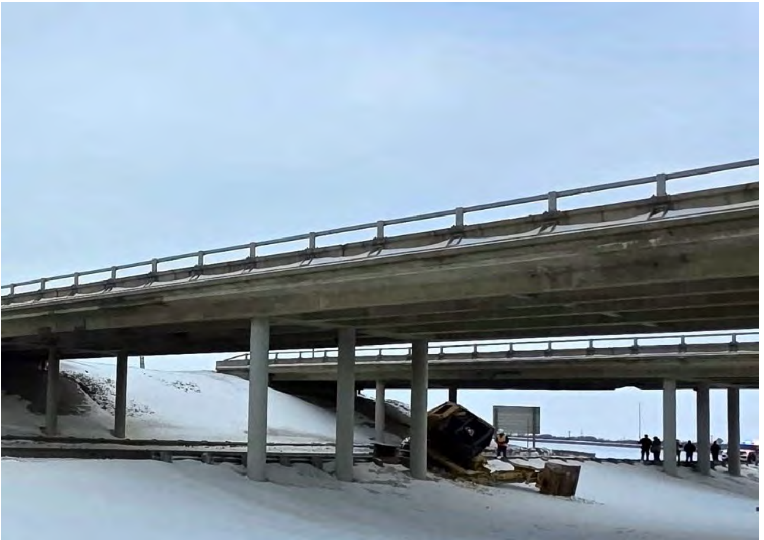
The other half of the excavator that hit the overpass. | Jon Perez
