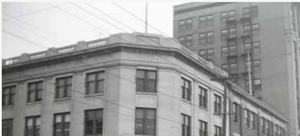
1962 Archival image of Credit Foncier Building, showing historical parapet construction with original balustrades
