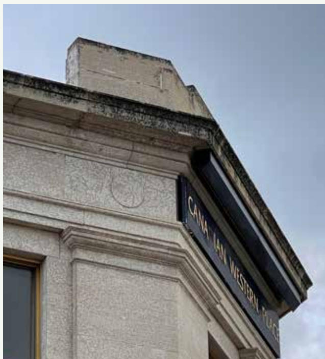
Credit Foncier Building, detail of the projecting Tyndall stone roof cornice and partial parapet, as viewed from the corner of Cornwall Street and 12th Avenue
