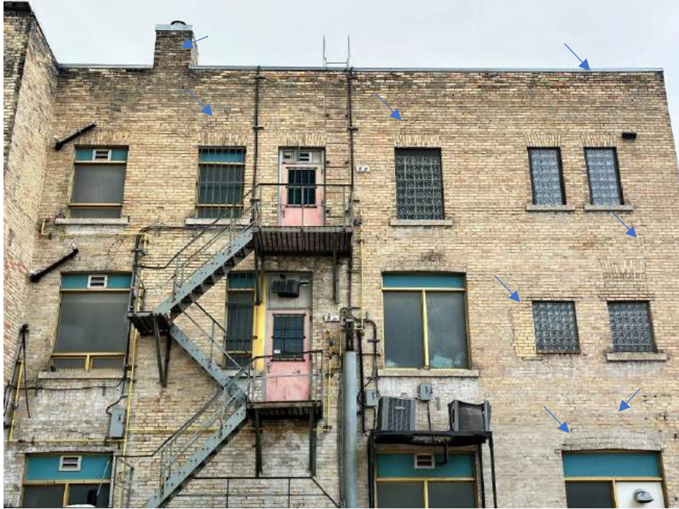
Photo 9: Cracks observed throughout the wall and eroded mortar joints the parapet
