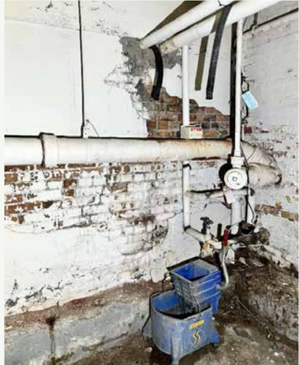
Views of the foundation wall where moisture had caused the surface to fail
