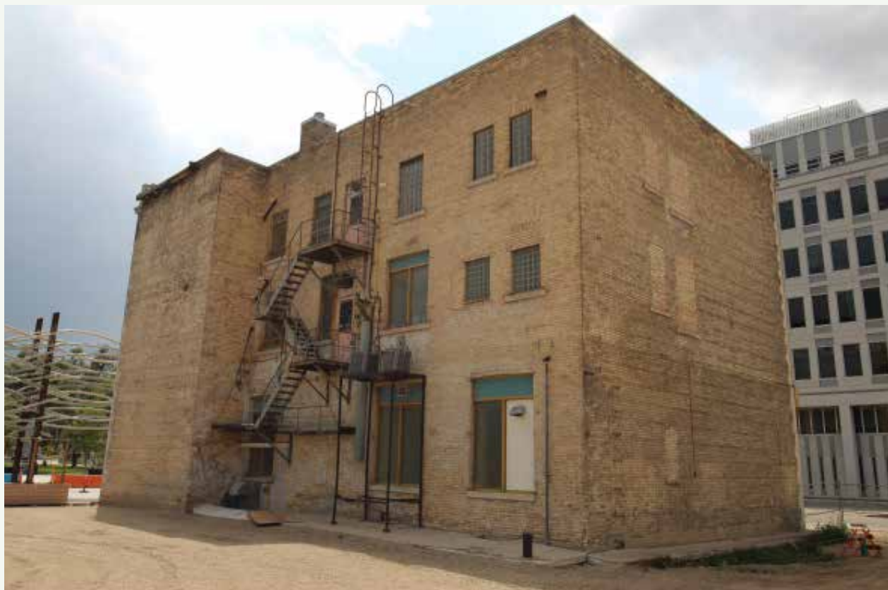
Rear brick façades showing blocked openings, fire escape, and mounted mechanical units
