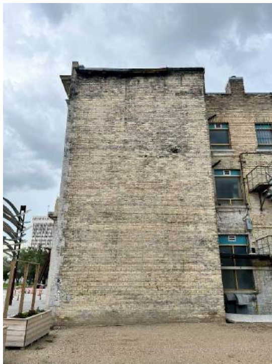
Photo 6: Partial View of the East Elevation
