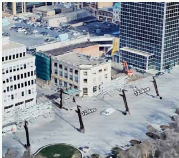
Aerial view of the Credit Foncier Building roof, showing the flat roof form and surrounding context (Google Earth)
