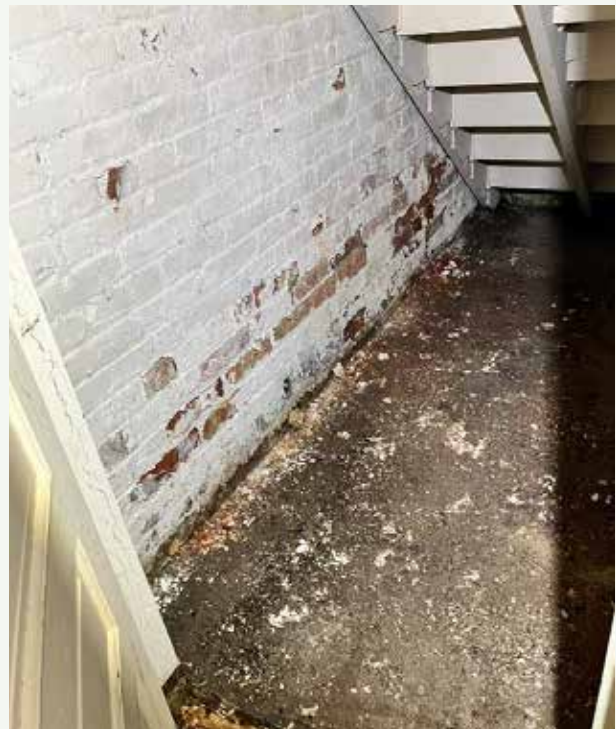
Views of the foundation wall where moisture had caused the surface to fail
