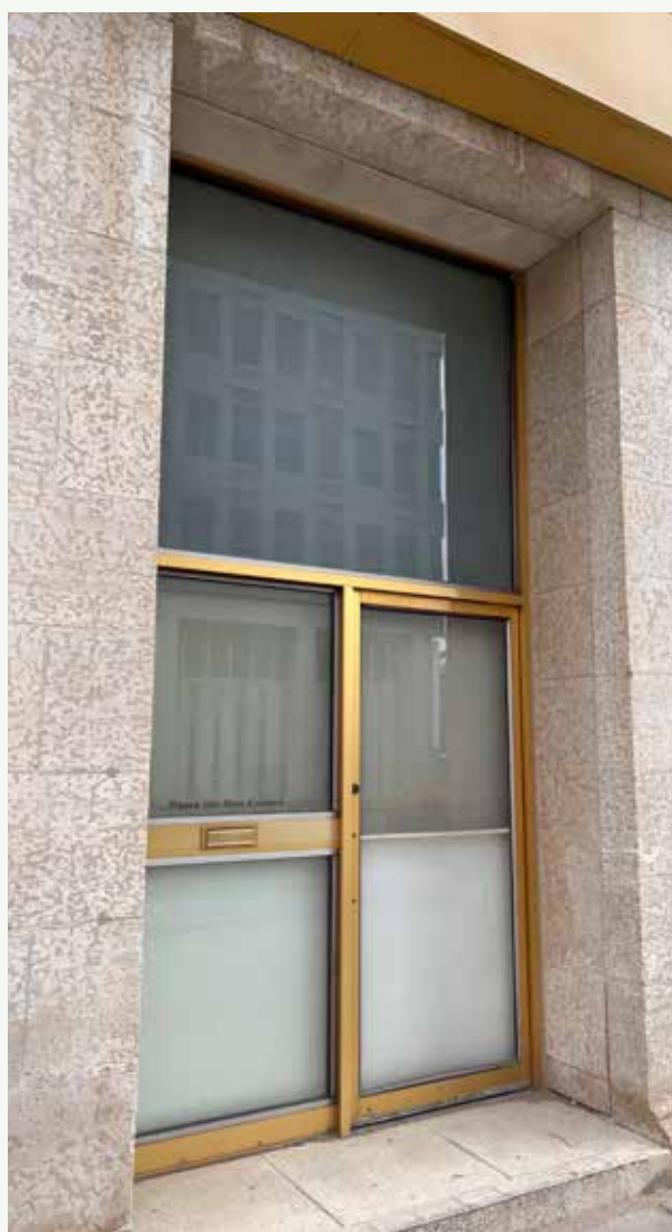
Original masonry opening at the north end of west façade facing Cornwall Street, with modern door and transom inserts
