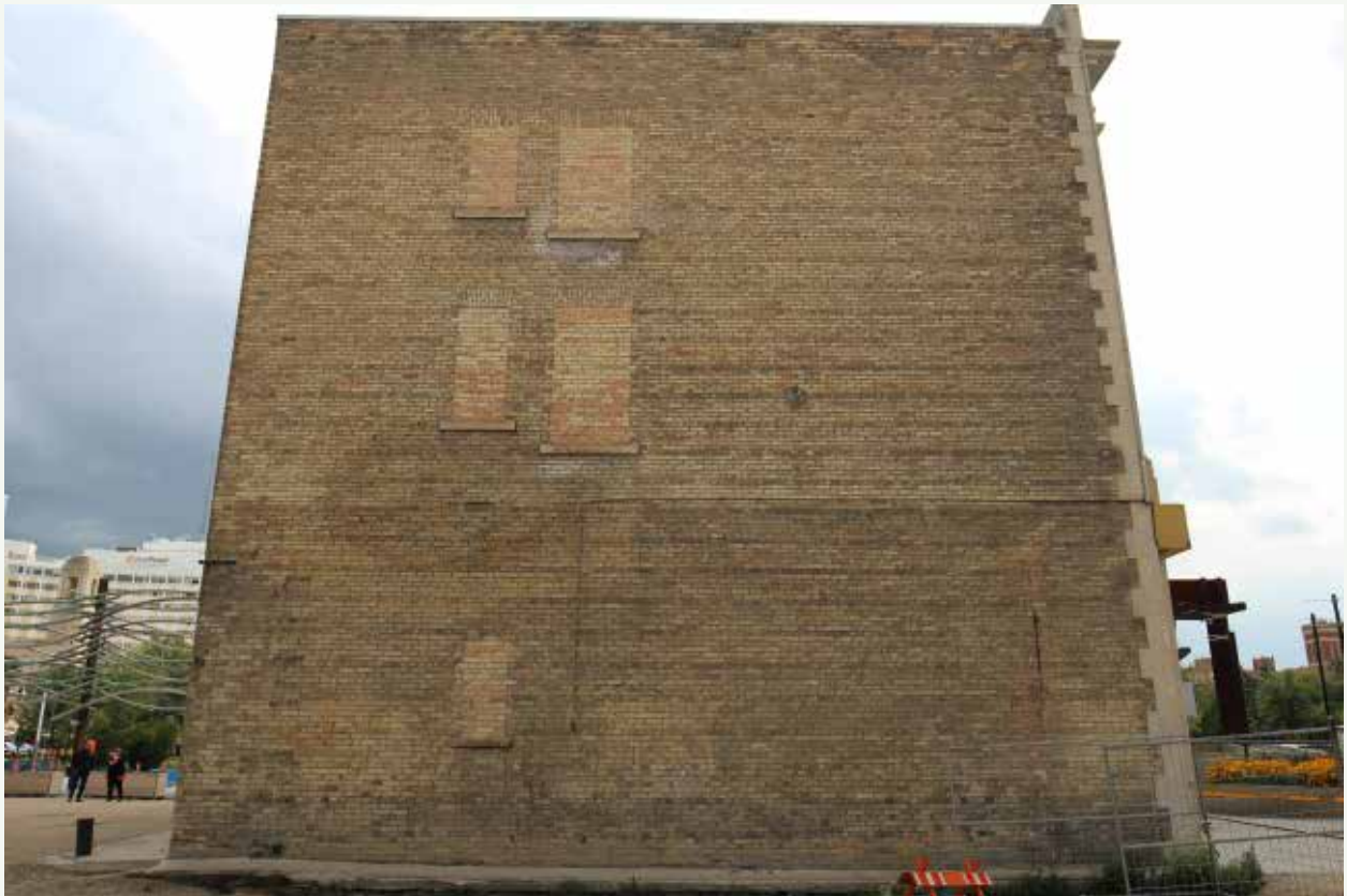
North brick façade with infilled window openings
