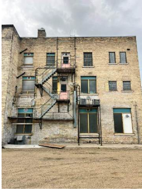
Photo 7: Partial View of the East Elevation
