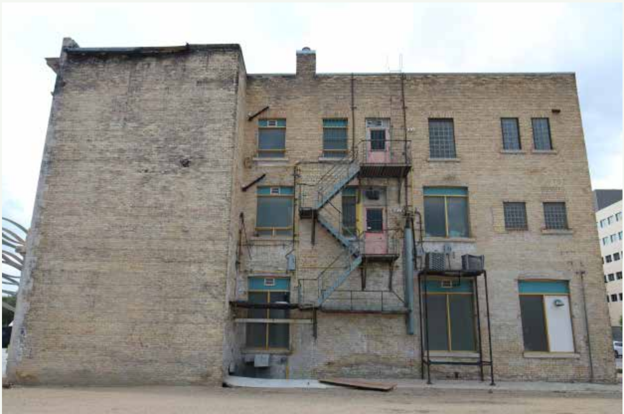
East brick façade with altered openings and fire escape
