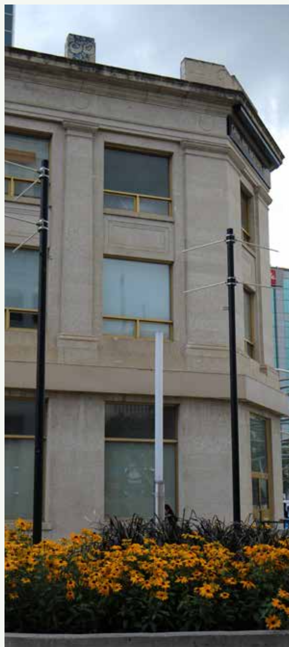
Detail of the Credit Foncier Building roofline, showing the flat roof assembly, projecting cornice, and parapet, as viewed from Cornwall Street
