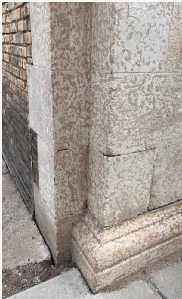
Corner condition showing Tyndall stone base courses and quoining detail, with adjacent brick masonry at return wall
