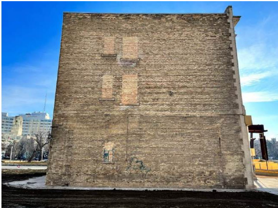
Photo 12: Elevation of the north side of the building
