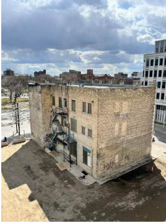
Photo 11: View of the building from the north east side of the building
